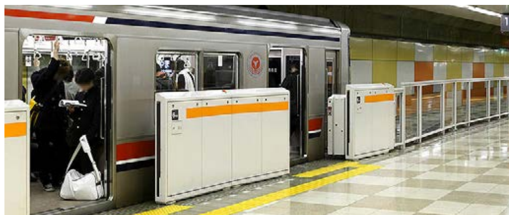
Platform screen doors of Ookayama Station, Tokyo Meguro Line
