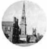
Landmarks are recognized and featured by view corridors and special lighting
