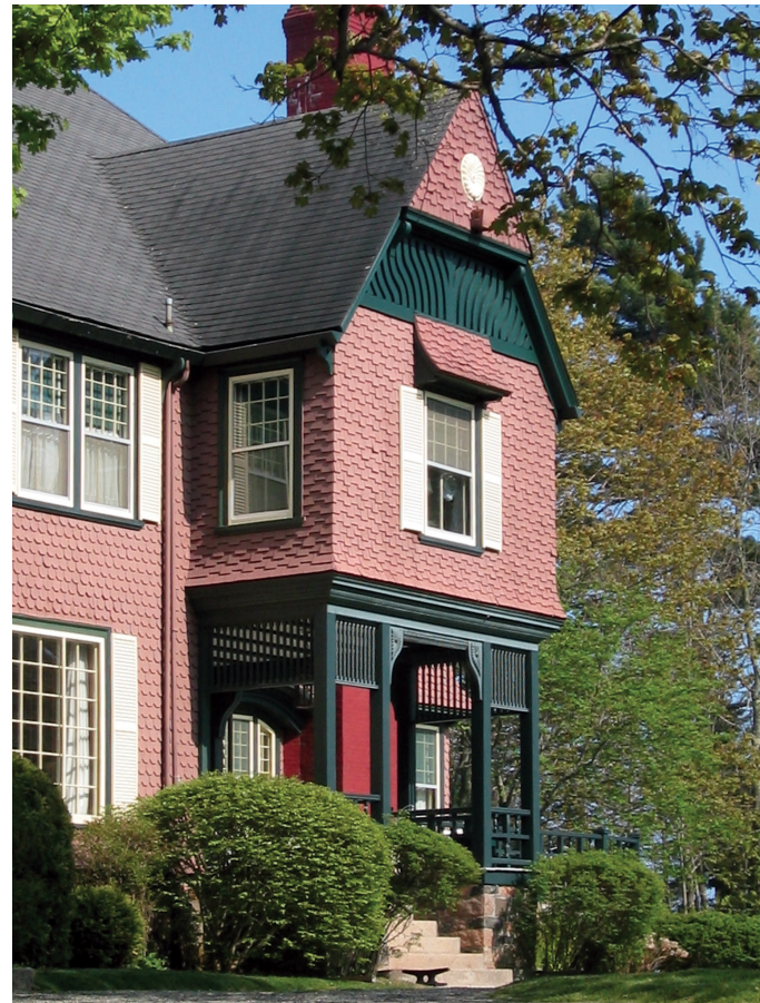
Fig. 7. Redwood, Bar Harbor, Maine, by William Ralph Emerson, 1879.
