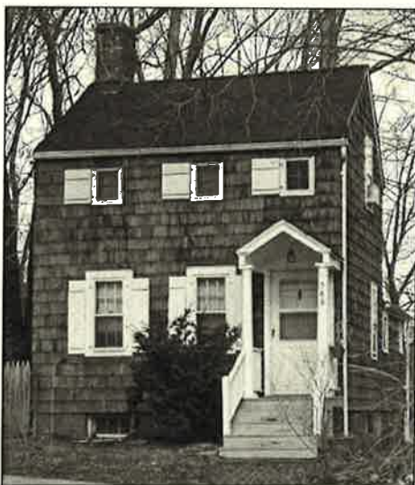
Howe house on Claremont Avenue in Montclair, once owned by former slaves James and Susan Howe. Photo by Mike Farrelly
