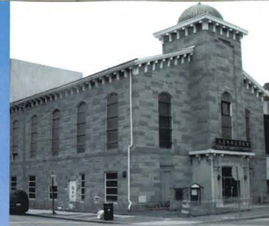
Built for a Presbyterian congregation in 1852, the restored sanctuary (left) is crowned by a replica of the original tower. Prior to restoration (above) the church was wrapped in cement Formstone.
