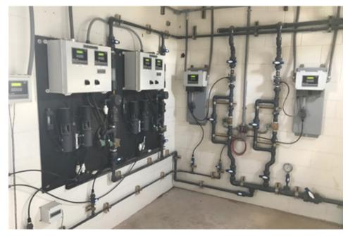
uses triple reversing servo motors coupled with v-notch valves to regulate the chemical feed rate, as well as an electronic flow sensor for the sodium chlorite, sodium hypochlorite, and hydrochloric acid. Both versions generate a more than 95 percent chlorine dioxide solution.
