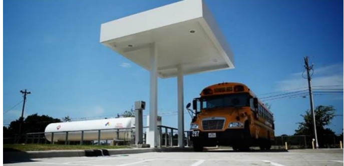
Figure 16: Propane autogas stations may be either private "behind-the-fence" facilities or public access like this station located adjacent to a school bus fleet, which serves as the anchor load.
