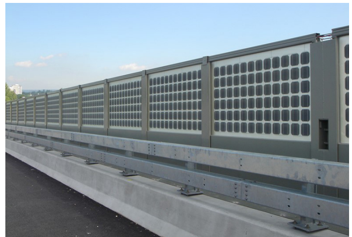
Figure 3. One of the first commercial applications of bifacial PV modules: noise barriers along roadways in Switzerland Source: TNC Consulting AG
