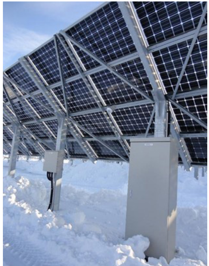
Figure 1. Example illustration of a bifacial system Source: Nikkei BP (Asahikawa Hokuto Solar Power Plant) Note: Picture taken from the rear side of an array of modules
