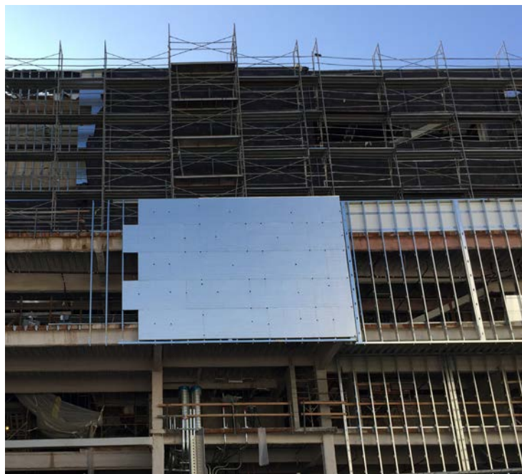
Steel stud construction with Rmax TSX-8500
