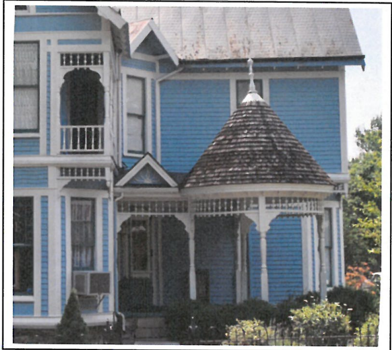
Elaborate porches, such as the one here at the Calvin House, are often important features of the Queen Anne style and should be maintained and preserved.
