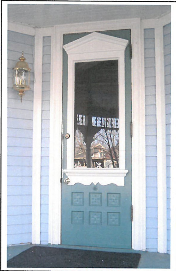
This elaborate door helps to define the character of this Queen Anne-style house and should be preserved.
