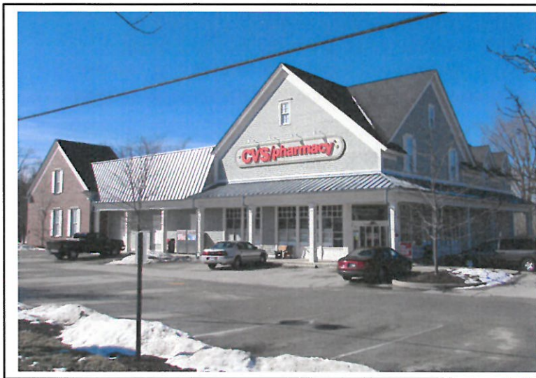
Different roof forms help to break up the massing of this building. Its unique design and use of traditional materials make it stand out from the chain retailer's typical stores.
