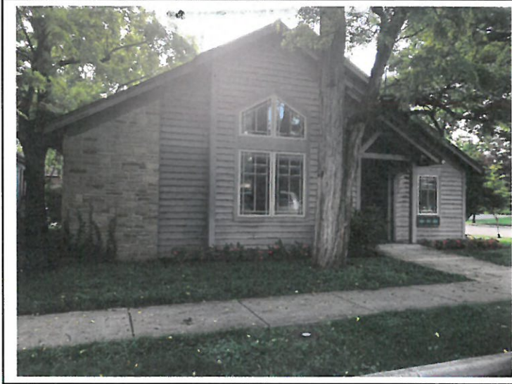
This office building is readily identifiable as modern, but the traditional materials and the pitch of the roof help it to fit in harmoniously with its older neighbors.
