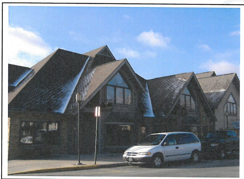
The complex roofline is an important character-defining feature of this building and should be maintained if alterations take place.
