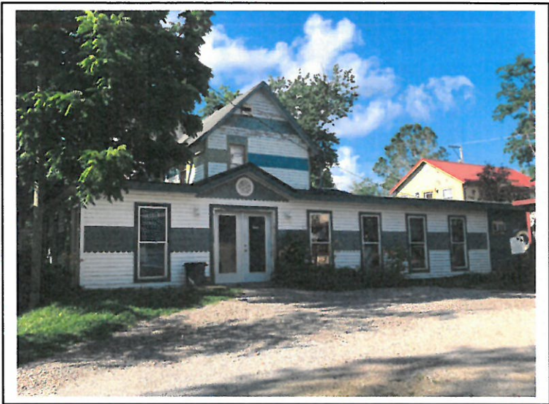
Although its orientation is much more horizontal than the house's, the use of similar siding materials and patterns, and the window shapes, help visually tie this addition to the main building.
