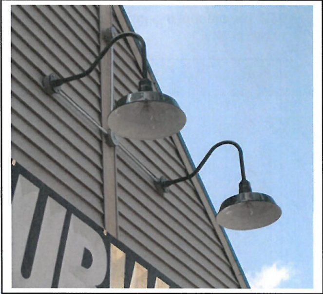
These gooseneck lights provide external illumination for the sign, as well as visual interest for the building.
