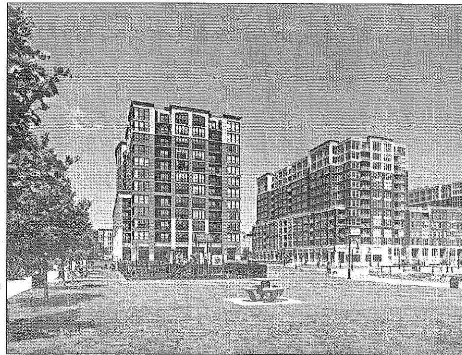
WORK IN PROGRESS – Two of the four development blocks At Maxwell Place are completed and occupied. The waterfront park, the restored beach, kayak pavilion, pier shed, and waterfront walkway are also completed and open to the community.
