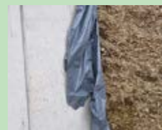
Lining the clamp walls with side sheets before filling the clamp is a key step to reducing air ingress.
