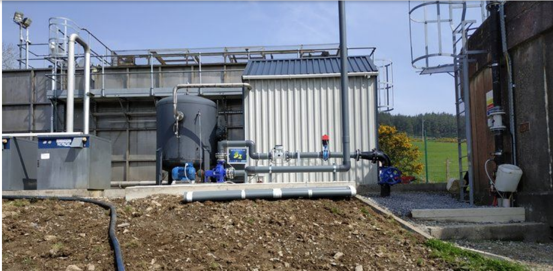
The low-cost and innovative pump-as-turbine technology at Blackstairs Group Water Scheme in Co. Wexford
