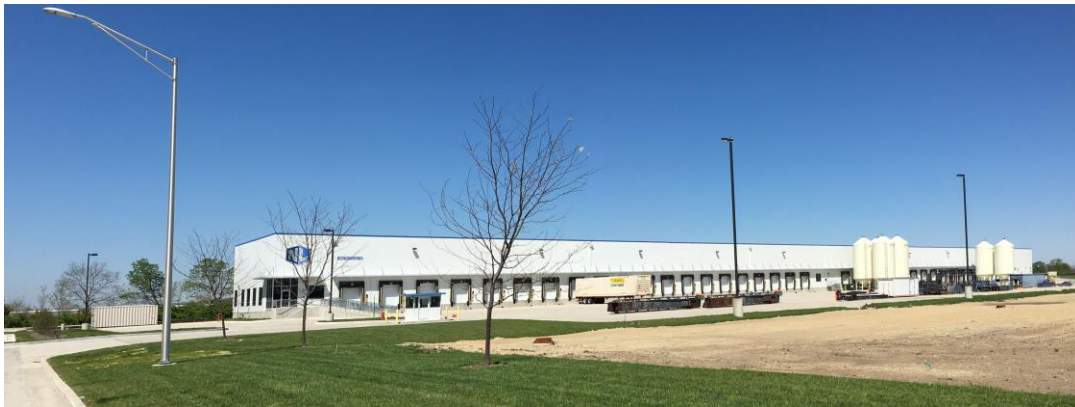
World Food Processing Refrigerated Warehouse
