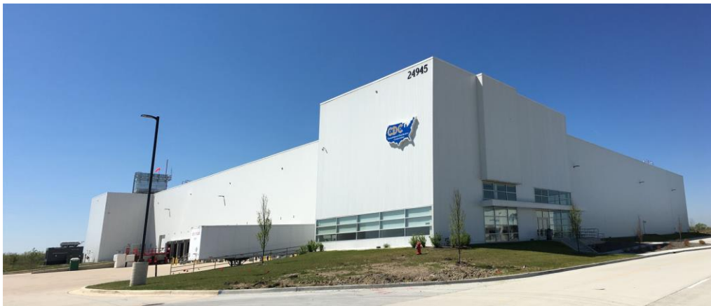
CDC Freezer Building
