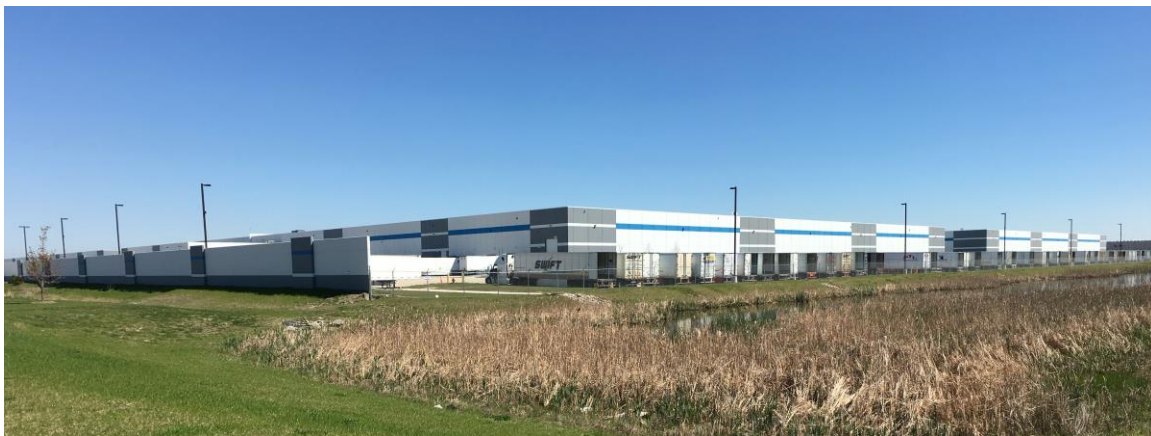
1,980,000 sq. ft. Michelin warehouse complex
