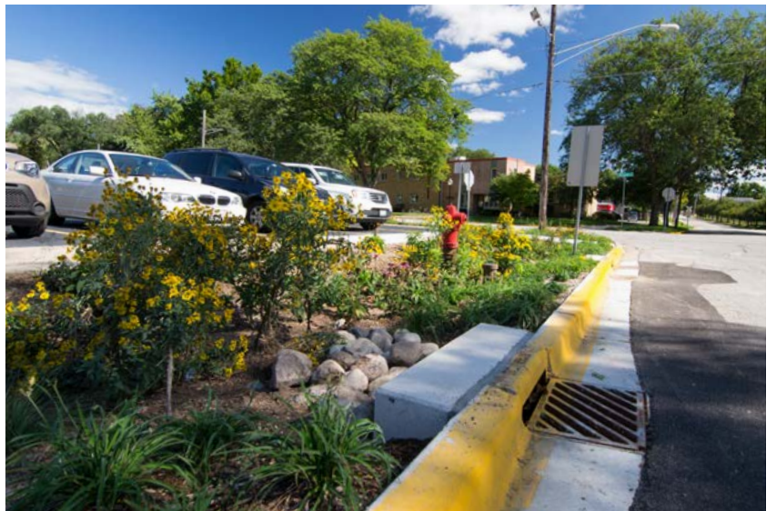
A series of rain gardens helps with surface runoff from the parking lot of Holy Angels in Aurora, IL. Source: RainReady: Center for Neighborhood Technology, 2017.
