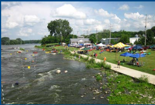
The Marge Cline Whitewater Park at Bicentennial Riverfront Park is a 1,100-foot-long bypass chute, built during reconstruction of the Glen D. Palmer Dam. The Illinois Whitewater Festival is held at this location in conjunction with Yorkville's annual Ribs on the River event.
