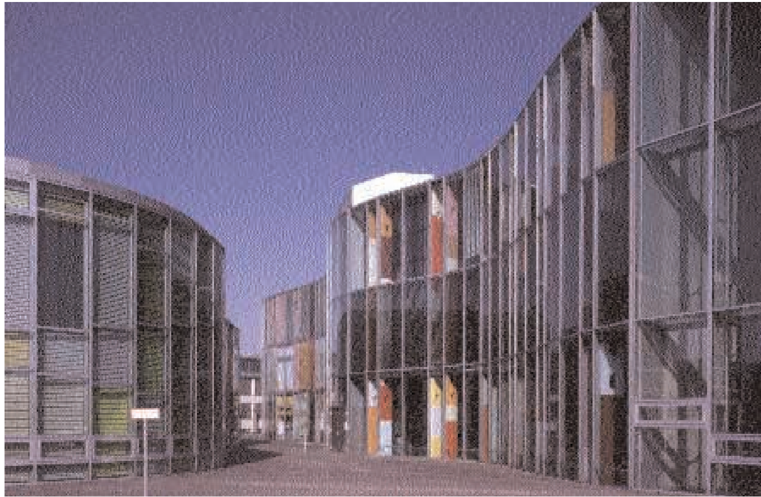
above: Pathway between the two blocks. facing page: Interior of the workshop hall. Exploded isometric sketch of the wall system.
