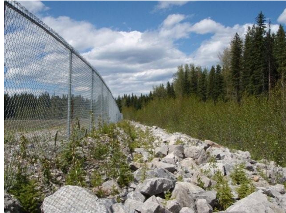
Flood protection at Elkford’s sewage lagoons
