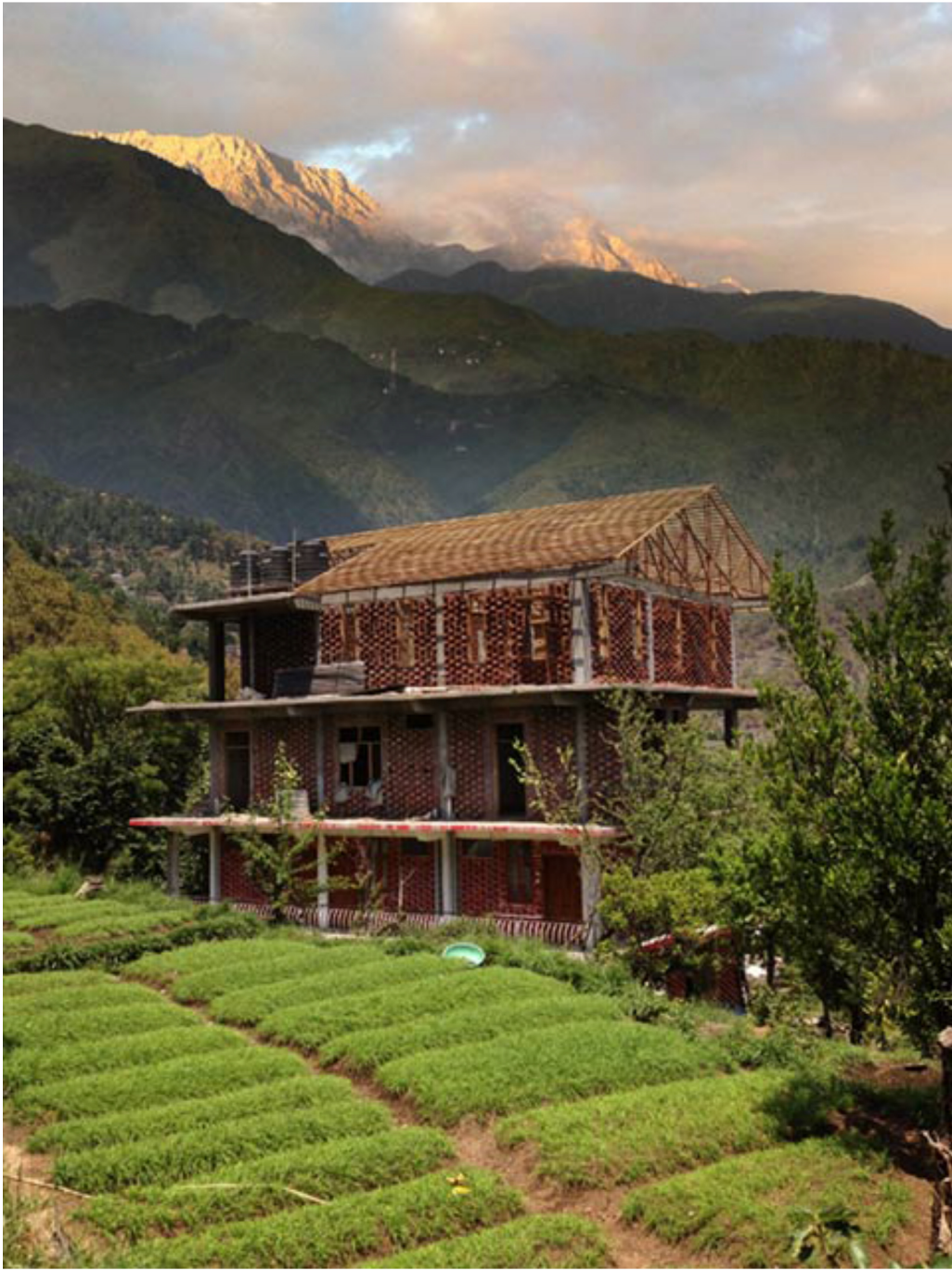
Himalayan Arts Centre under construction.
