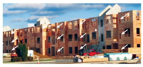
Multi-Family Construction utilizing **Comfort Pack** "Thru-the-Wall" units
