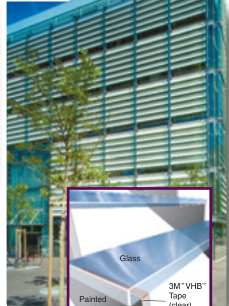
Glass steps bonded to varnished steel frame, Tamedia Building, Zurich, Switzerland
