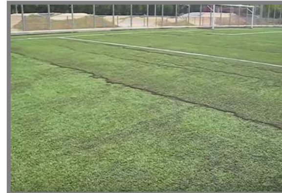
“Six-month-old synthetic turf field with Geo infill made of coconut peet after rain storm, Italy, 2009
