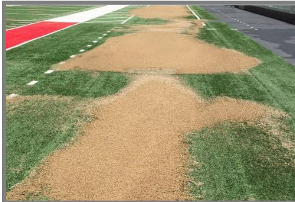
“This is what happens to cork infill after you get 2” of rain in 20 min! #itfloats #syntheticturf #fieldexperts ”
