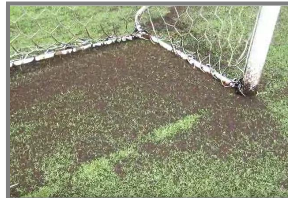
“Second field synthetic turf field, no longer playable, requires complete refurbishing after same rain storm ”
