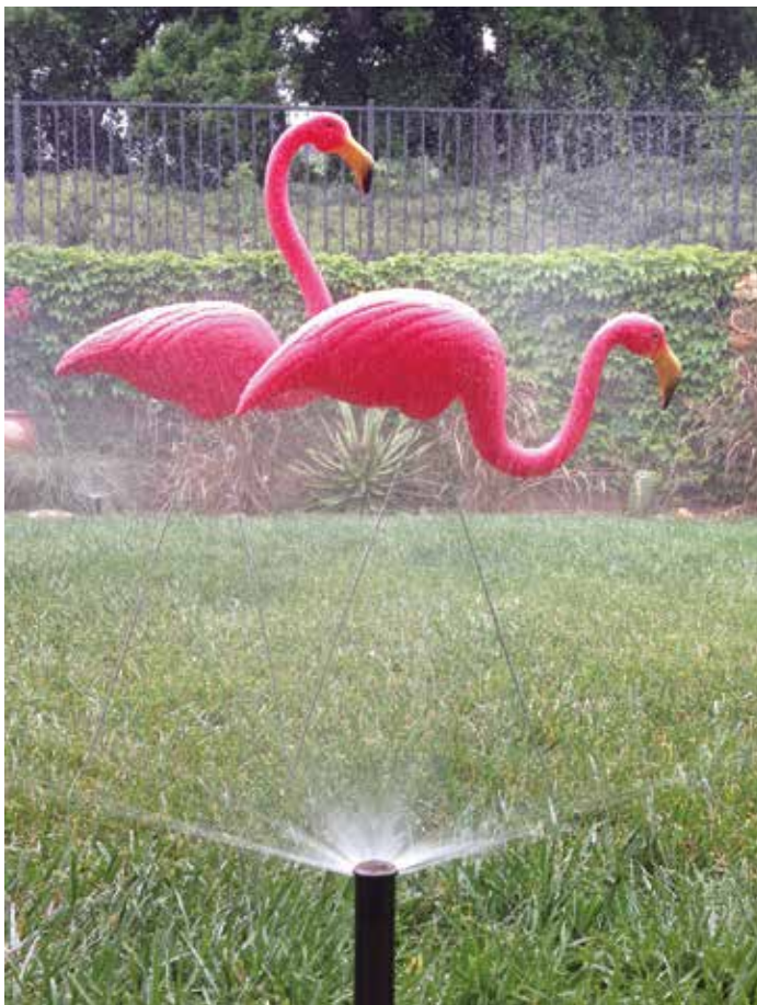
IMPROPER INSTALLATION – No flexibility
