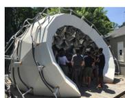
Comprised of 9 parts robotically cut foam, 2 parts gorilla glue, 1 part mylar, and many parts thermodynamic theorizing, CHAOS Lab presented their foray in indirect evaporative radiant cooling on September 1, 2014. The ThermoHelioDome combines a cooling tower and spherical and conical geometries to focus the effects of evaporative cooling on the interior of the spherical dome shape by focusing the radiation from the cooled bulbs on occupants. [[chaos.princeton.edu](http://chaos.princeton.edu)]
