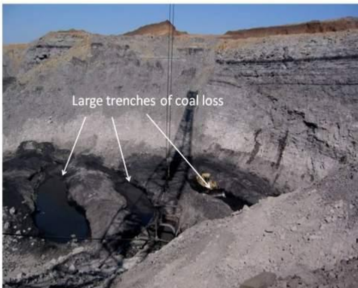
FIG 11 - Coal loss with the formation of deep trenches, despite use of buffering and baby decks
