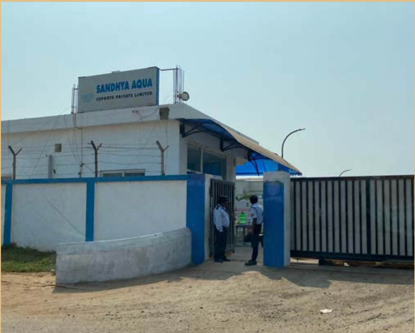
A Sandhya Aqua processing plant (Andhra Pradesh, 2024)
