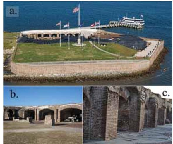
Figure 1: The current state of Fort Sumter National Monument: (a) aerial view, (b) barrel vaulted casemates, and (c) degradation of brick and mortar piers.
