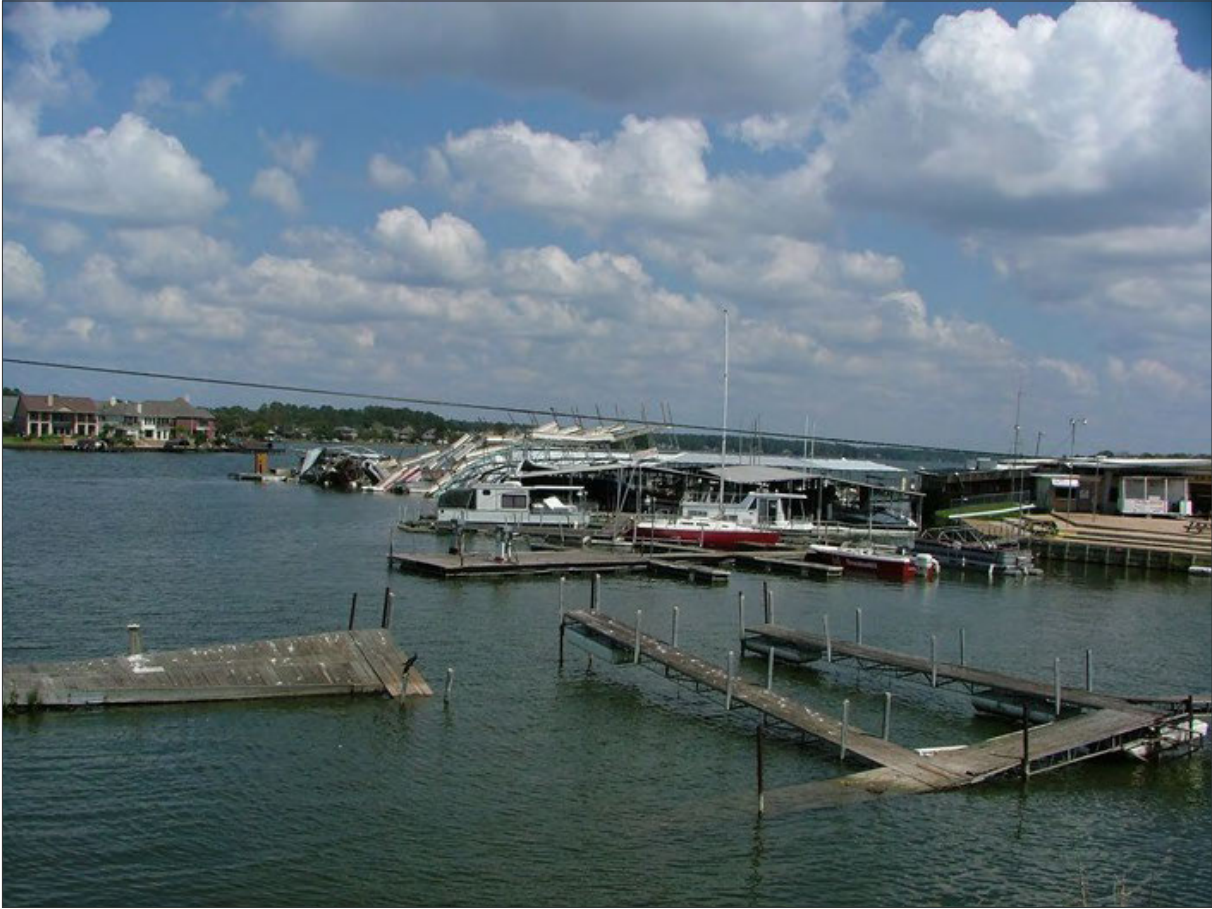
Hurricane Ike Storm damage at Lake Conroe boat ramps
