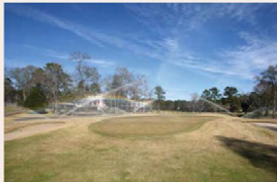
Photo 6: Application. Treated water is pumped from the holding pond by high pressure pumps to the sprinkler system.
