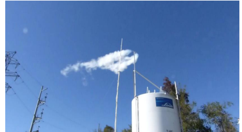
LH2 Venting following delivery
