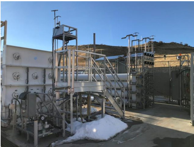
The LRQA installed on HITRF
