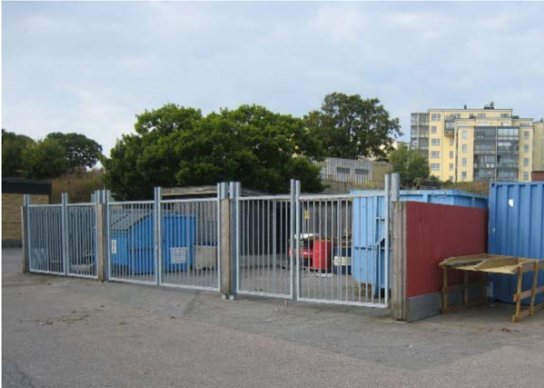
A fenced waste collection site at the harbour of Saltö, Karlskrona.
