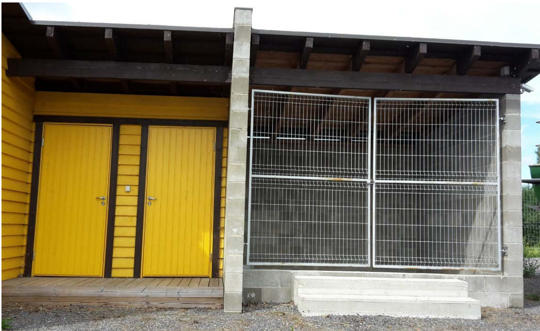
A port must have a separate lockable room or a fenced area in its territory for the collection of bulky waste. The photograph depicts a storage room for bulky items, including waste, at the harbour of Lindi.
