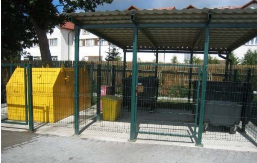
A modern waste collection station at the Port of Dziwnów. The new waste station is mainly targeted at the tourists visiting the yacht harbour.
