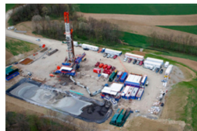
Figure 12- Fracking site with wastewater storage pit
