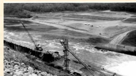
The Dam under construction
