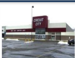
Flint Strip Center 4071 Miller Rd. Flint Township, MI Retail Strip Center
