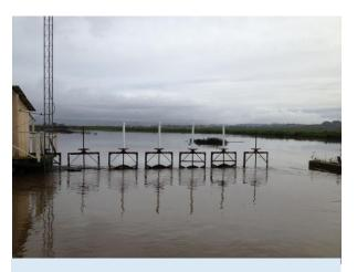
Figure 6. Tide gates at Watsonville Slough flooded during a January 2017 king tide.
