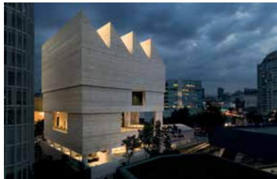
Museo Jumex in Mexico City, by David Chipperfield Architects
