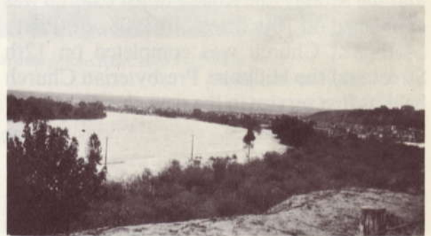
Flood scene of Sunnyside.
