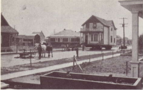
One of several houses moved to make room for the Sunnyside Elementary School, 7th Street and 2nd Avenue. Heading along 1st Avenue, the house is being moved by horse and platform, circa 1921
