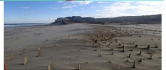
Laminar flow encountering turbulence will drop sand.
