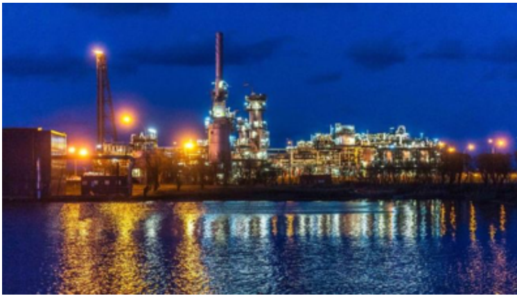
The St Fergus Gas Terminal is involved in the Acorn Project. Photo credit: North Sea Midstream Partners
