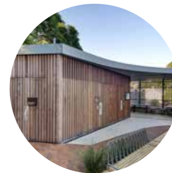
New Toilet Facilities
