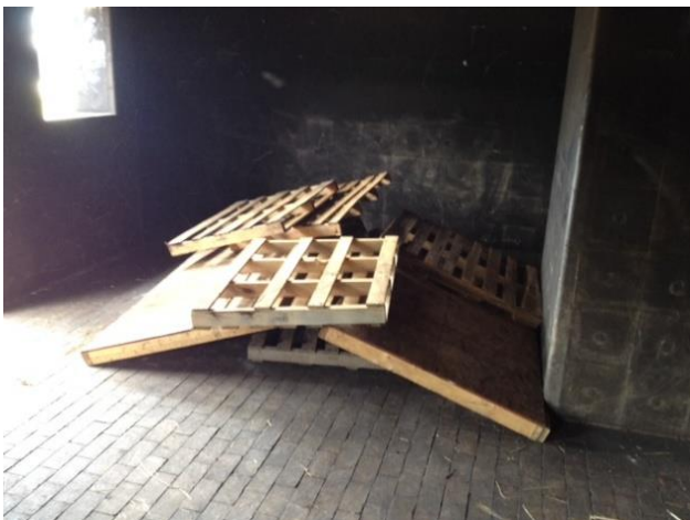
Figure 5: Complete debris pile on top of compromised firefighter
