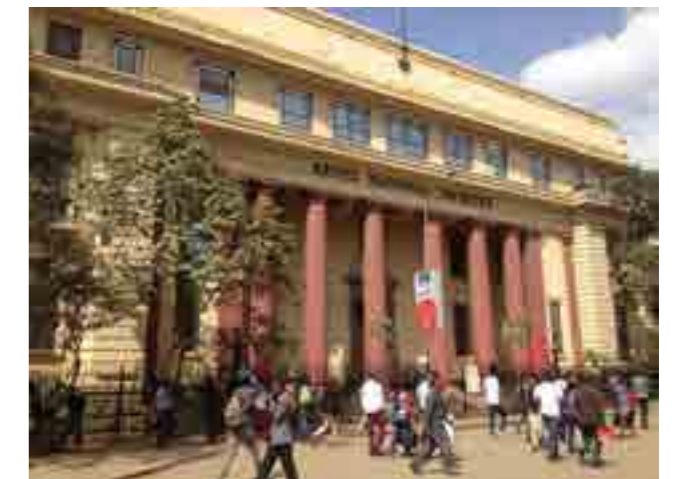
Building of National Archives of Kenya, Nairobi. Photo: Marian Nur Goni
