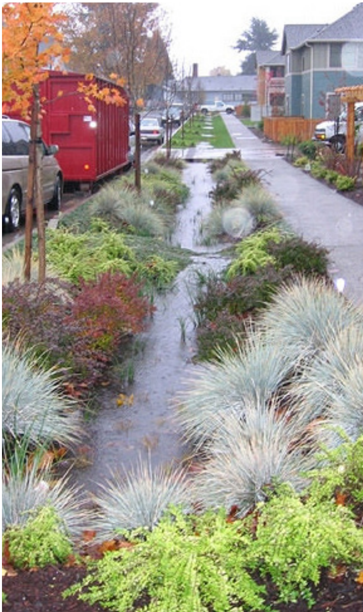
An example of a rain garden used to manage stormwater runoff in a residential area. Photo: US EPA
