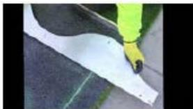
Super Seamer Tool: This S-shaped tool creates a smooth surface that makes turf easy to seam pieces together. It alleviates the common synthetic turf "Mohawk effect" in four easy steps.
