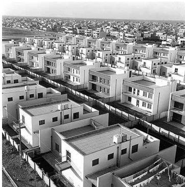
Figure 2.2. Housing Project, Mamoun District, Baghdad, 1960. Latif al Ani Collection (Copyright, Arab Image Foundation)
