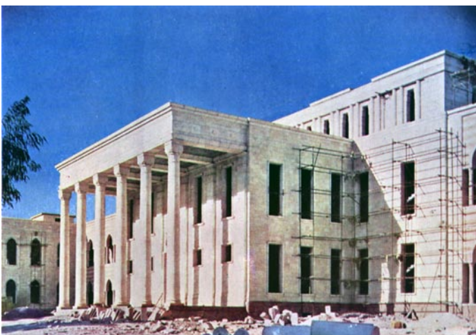
Figure 1.6. The New Iraqi Parliament Building, under Construction in 1957
