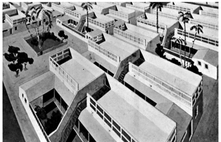
Figure 1.12. Housing Project Planned by the Development Board, Published in the 1957 Development Week Pamphlet without Reference to Its Well-known Designer, Greek Architect Constantine Doxiadis
