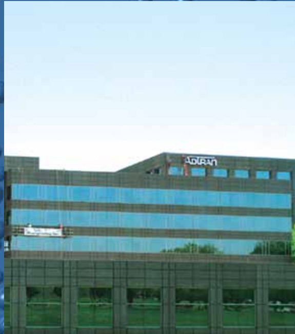
Caulking & Wet Glazing Windows and Window Washing
