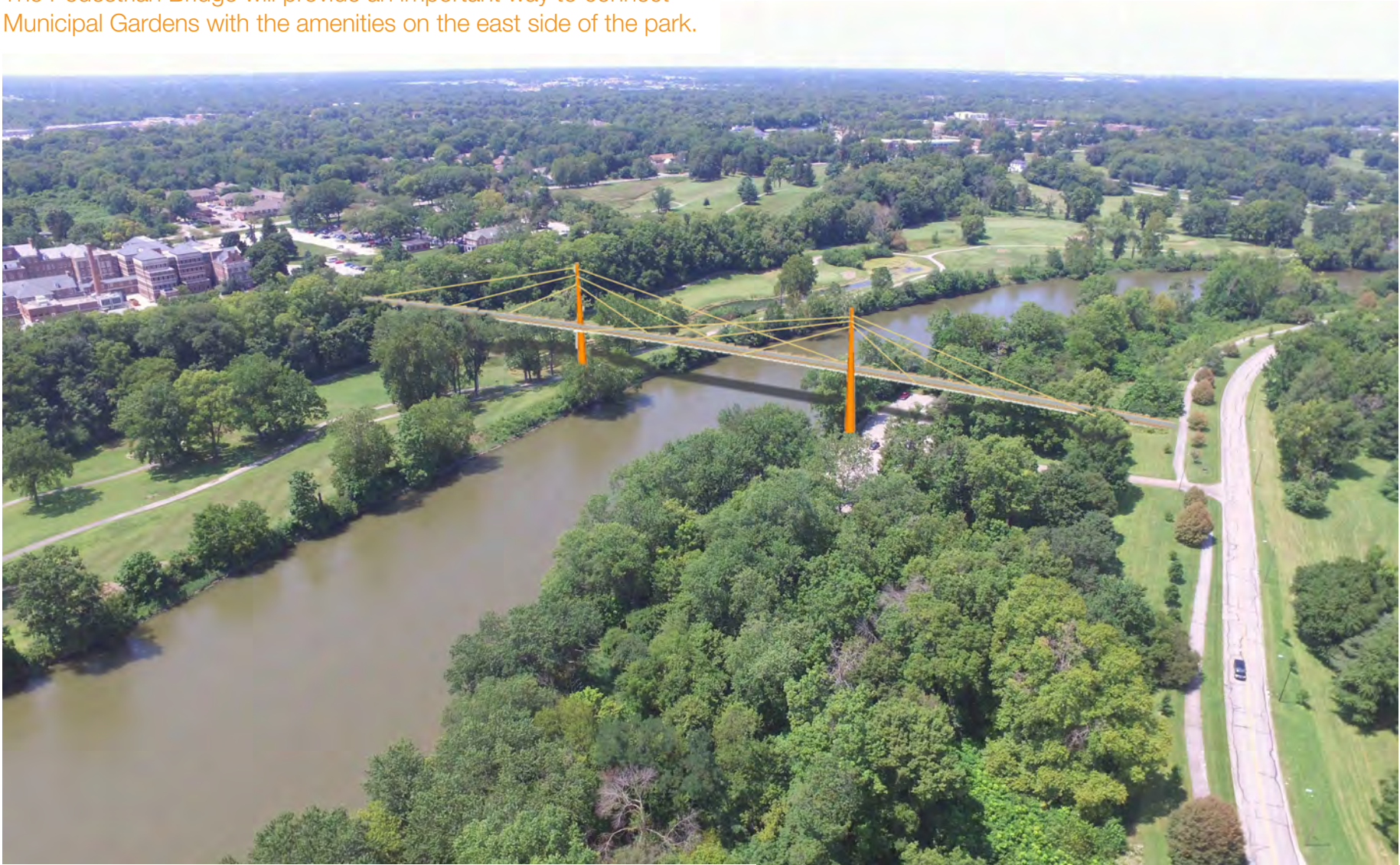
Pedestrian bridge spanning the White River from Lake Indy Boat Launch to Larue Carter Memorial Hospital
