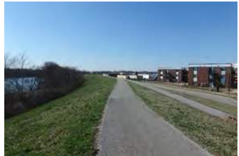
Levee WR-20 South of Riverside Regional Park
