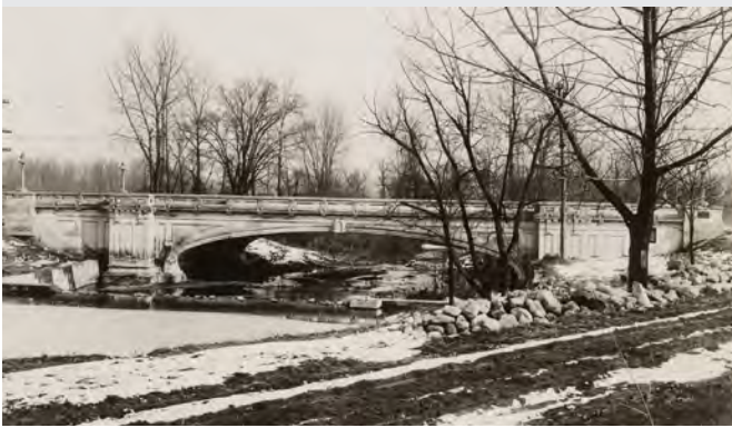
Cold Spring Road Bridge at Lake Sullivan
