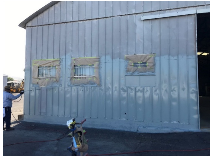
Lindsay maintenance staff painting the Lindsay yard buildings
