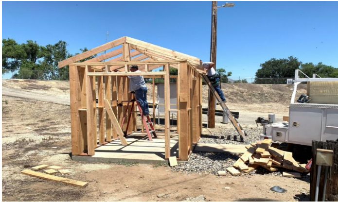
Orange Cove maintenance staff constructing generator shed at Kings River Check
