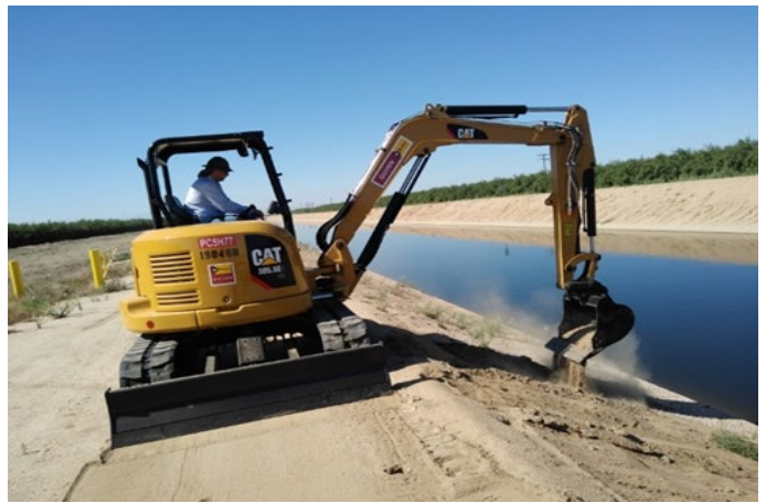
Delano maintenance staff continues embankment maintenance
