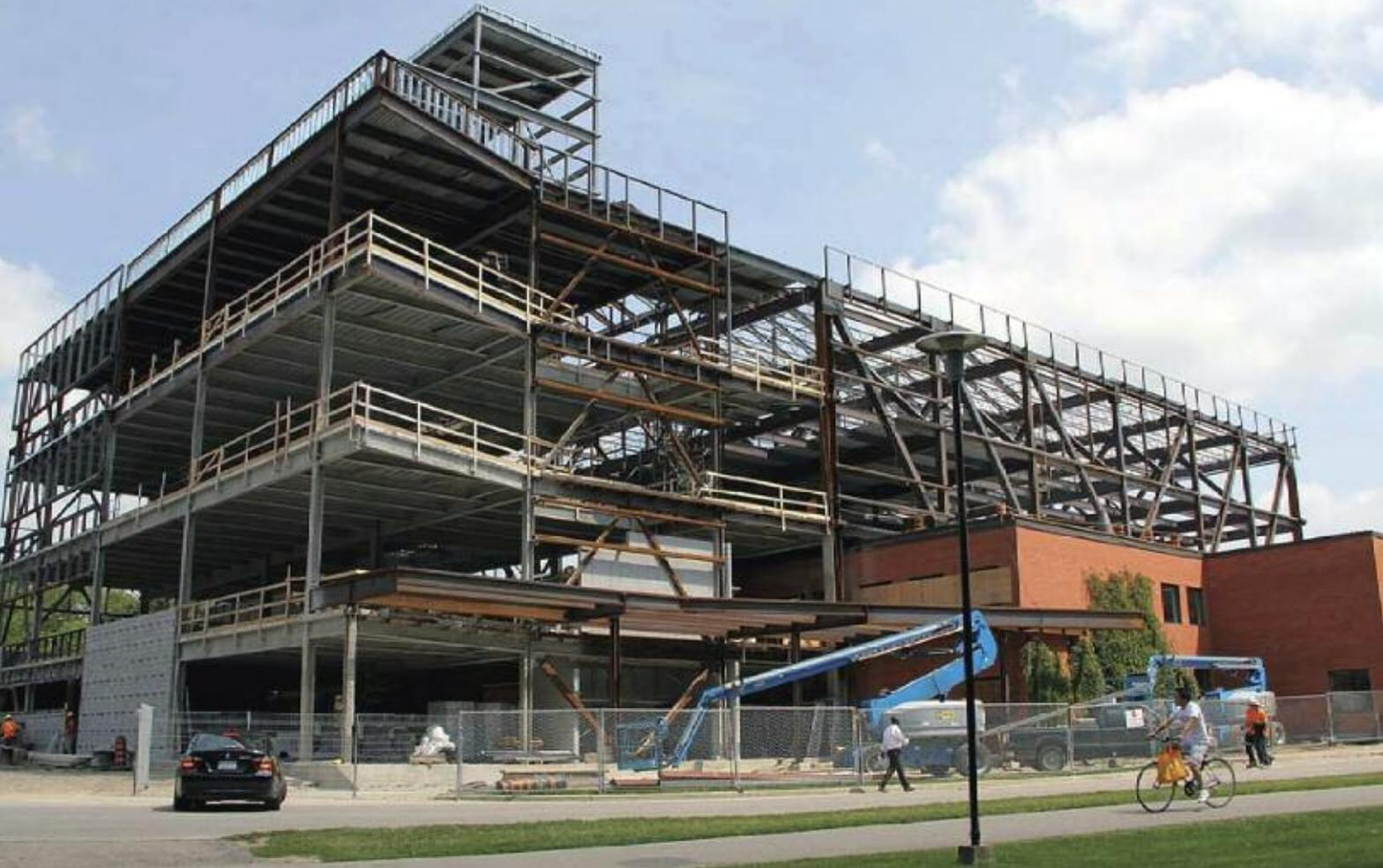
Two large 2-storey 10m high x 47m long (32.8 ft. high x 154 ft. long) steel trusses form the sides of the 3rd and 4th floor addition and are supported on columns located clear of each end of the EV2.
