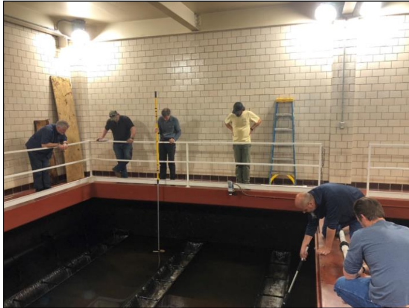
FIGURE 20. Filter No. 1 media expansion determination.
