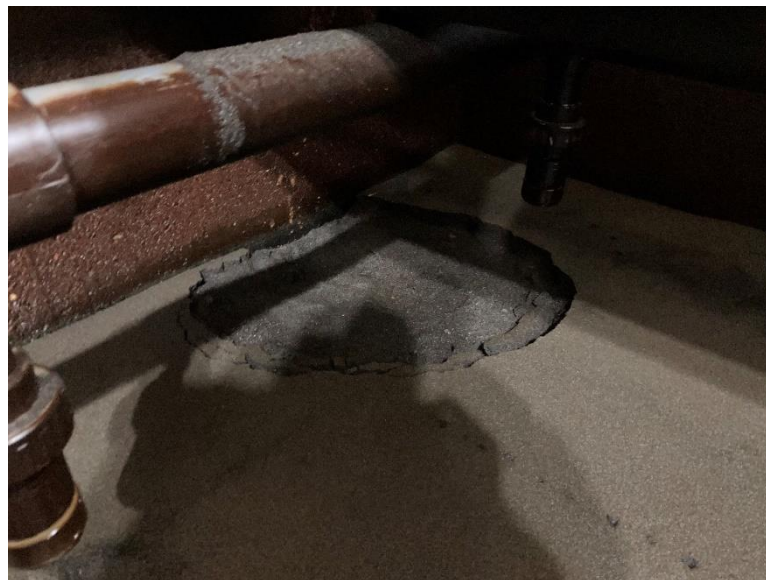
FIGURE 17. Cratered area in Filter No. 1.
